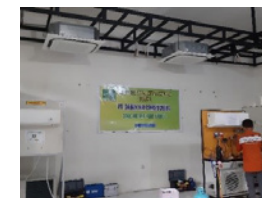
PT. Daikin Airconditioning Indonesia Provided equipment to technical school
