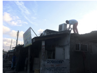
Installing an outdoor unit on a house
