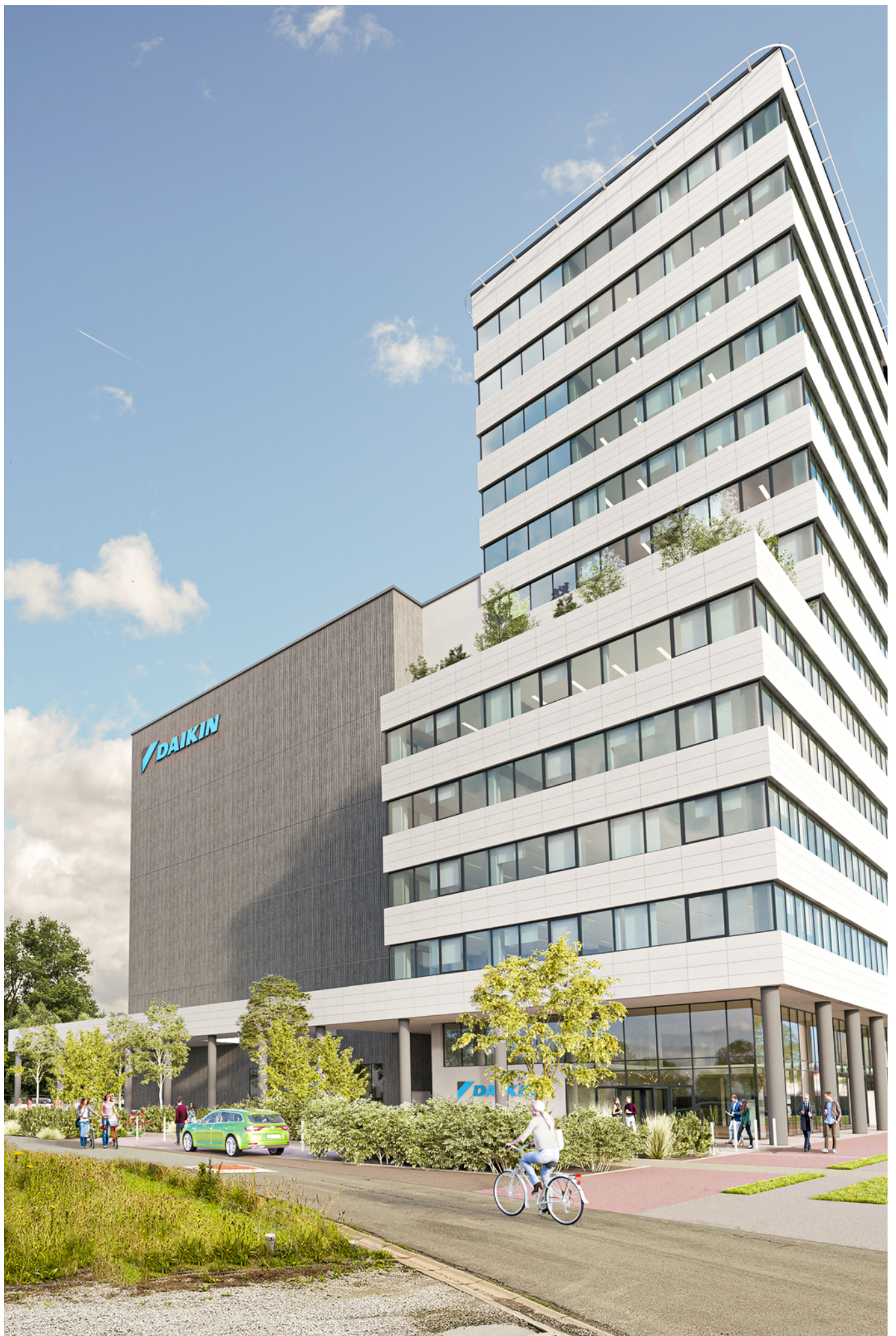
Daikin Europe Research and Development Center - 11,000m 2 Testing facilities & 10,200m 2 office space.
